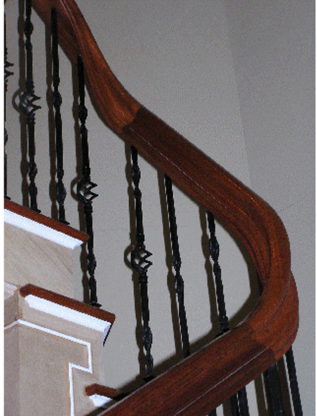
Handrails machined with VisualMill 4th and 5th Axis modules
